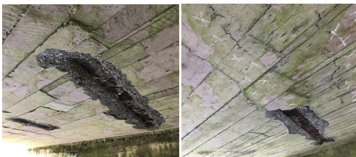
Figure 3-1 - Spalling and exposed filler beams evident to both the south span (L) and north span (R)
